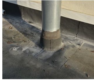
Penetrations/cracking
